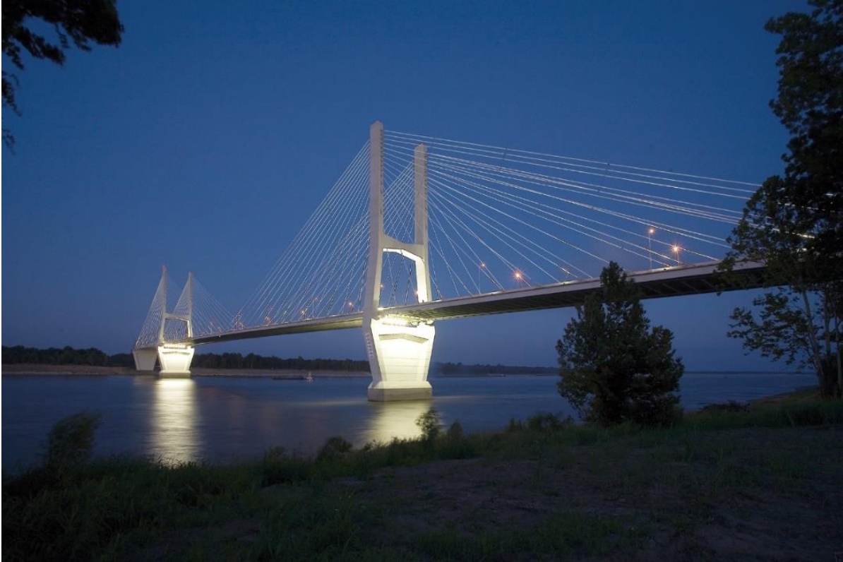
Greenville Bridge: ST delivers cable-stayed bridge construction support
